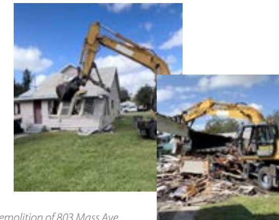
Demolition of 803 Mass Ave
