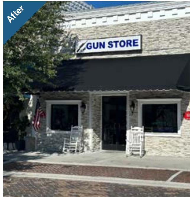
Building and Site Improvement Grant (BSIG) Program storefront after improvements
