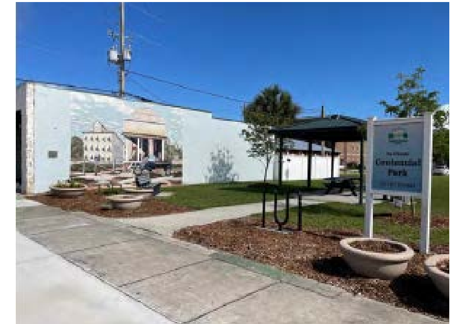
Centennial Park Improvements
