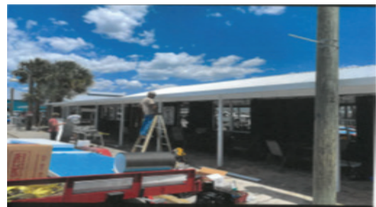
The Salty Hobo - New front porch for additional seating $6,700
