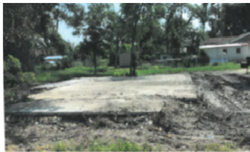
Alto Thomas - Demolition $1,250
