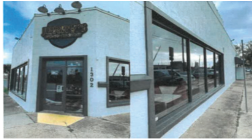
Jerry's Burger - Clean, repair, and paint exterior $1,900
