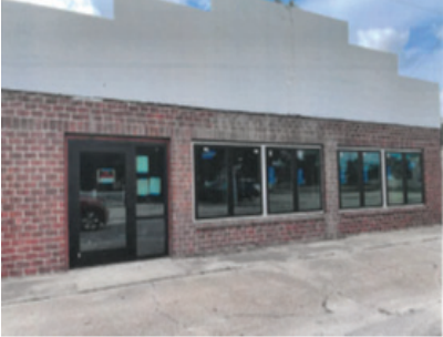
611 Mercer Dr - Roof, Windows and doors $50,000
