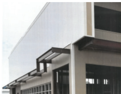
McLeod's Glass & Supply - Roof deck & exterior walls $50,000
