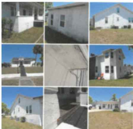
Bishop Johnny & Shirley Wayde - Repairs to front porch and chimney $8,577.50. (before photo)
