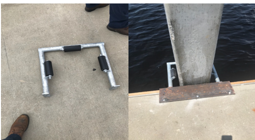
St. Andrews Marina - Floating dock repair
