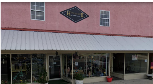
1105-1111 Beck Ave - New roof $22,500
