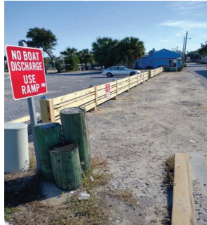
Bayview & 11th Ct - Fence installation
