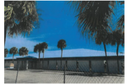
The Clinic Building - New roof $50,000
