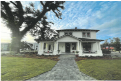
The Sapp House - Landscaping & hardscapes $24,620.47
