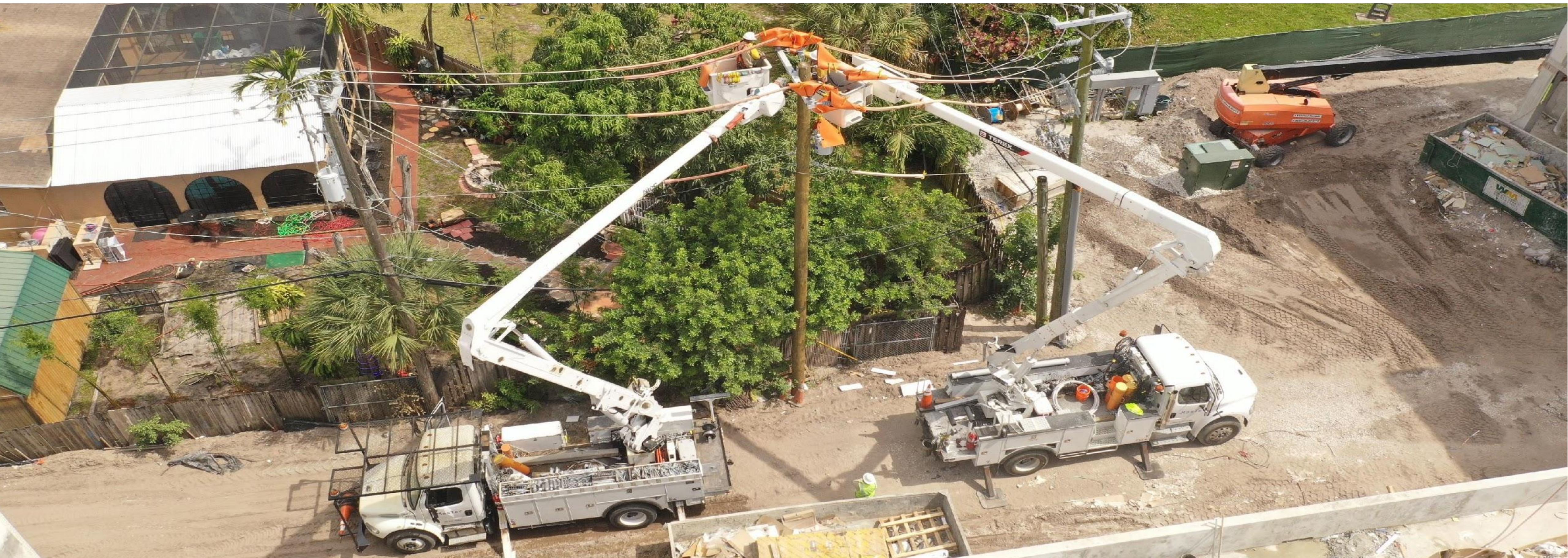
Undergrounding overhead utility lines.
