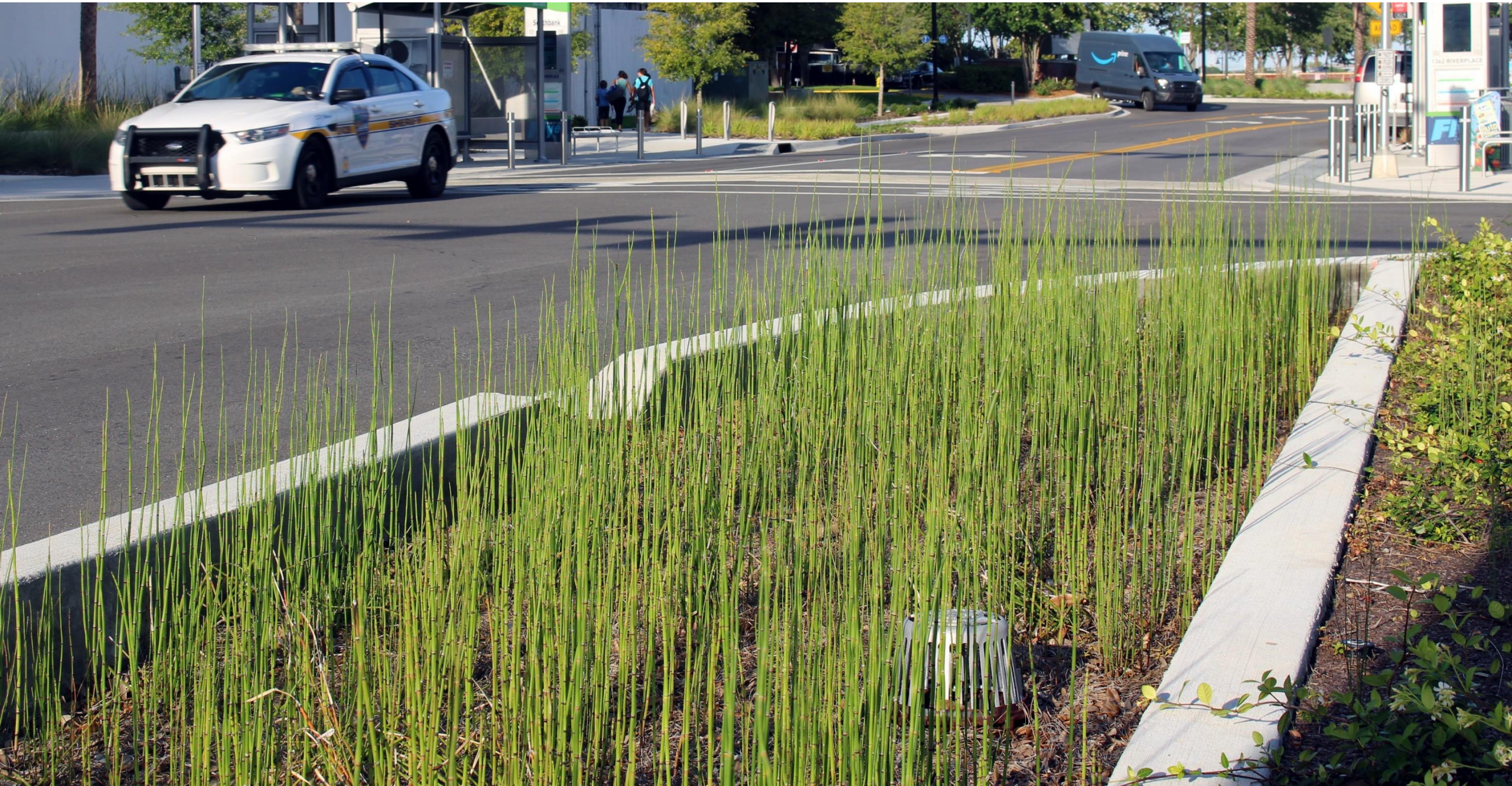
Image #12: Detail of typical rain garden with open curb drainage flume to recessed planting area (Juncus) & overflow inlet.
