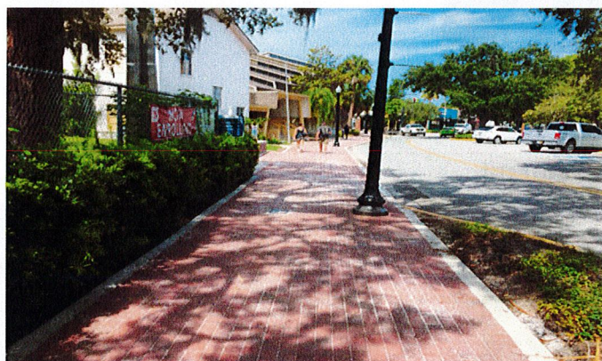
Paver Replacement Project
