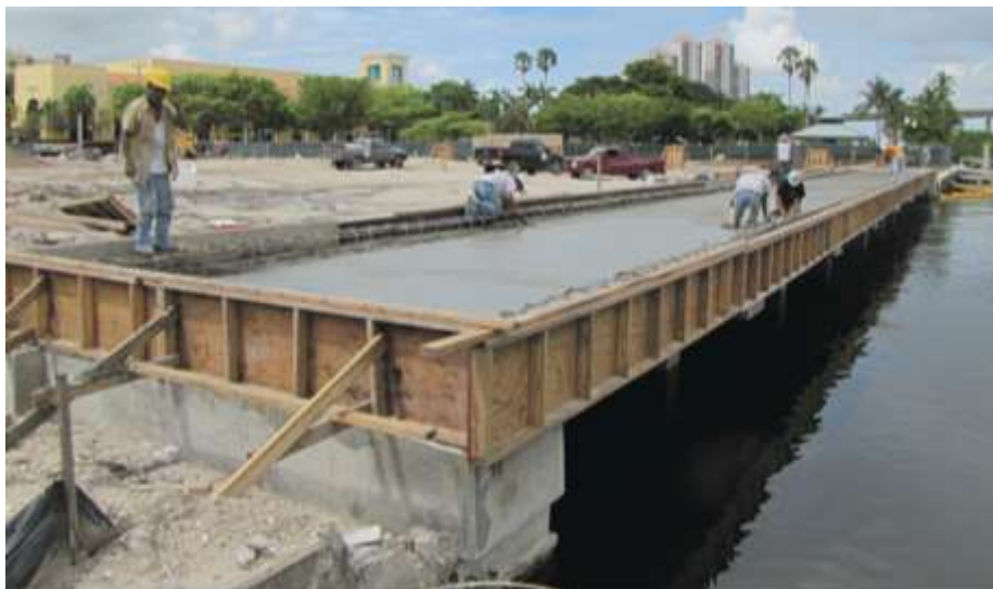
Constructing the “floating” walkway over the weir.
