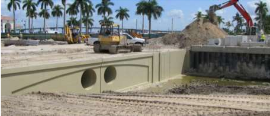
Basin is sloped to provide a littoral planting shelf
