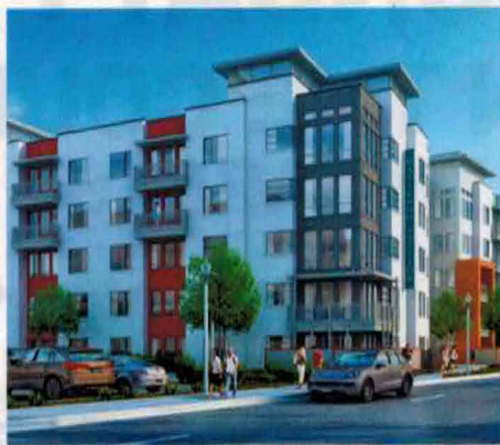
▶ Maitland Station will go up on land formerly owned by Parker Lumber.
