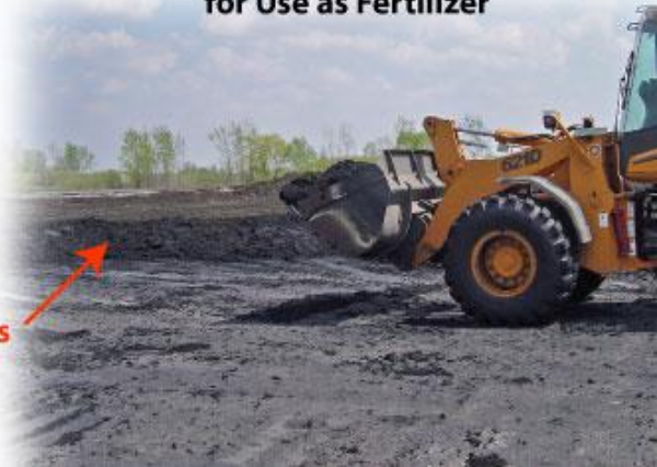
A Biosolids Holding Area Where Biosolids are Loaded onto Dump Trucks to be Transported to Agricultural Fields for Use as Fertilizer
